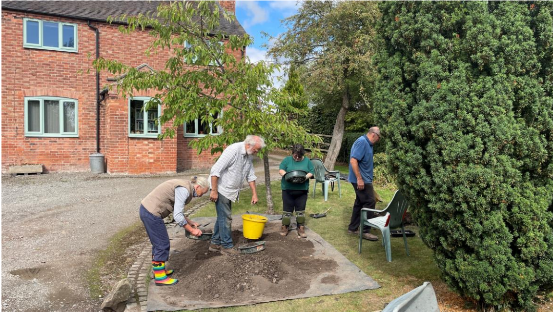
Figure 11: Test Pit 4 during excavation. Looking north
